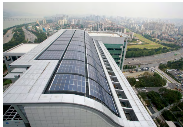
Smart Solar Solutions installed at Seoul Asan Medical Center
